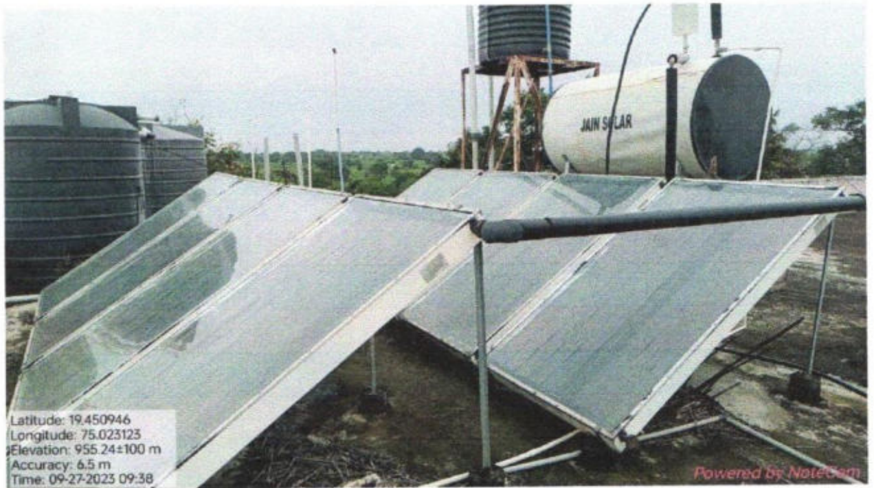
Jain Solar Water Heater System, close Loop 1000 LPD
