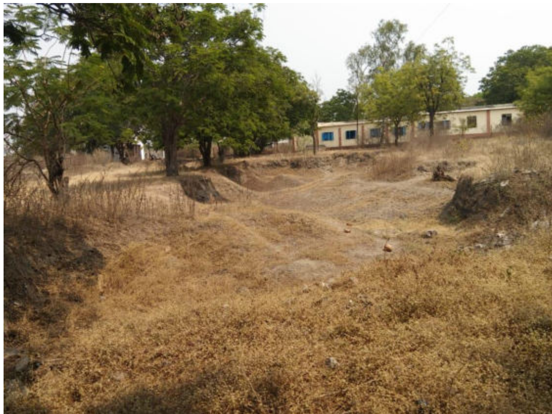
Natural Pond for Rain Water Storage
