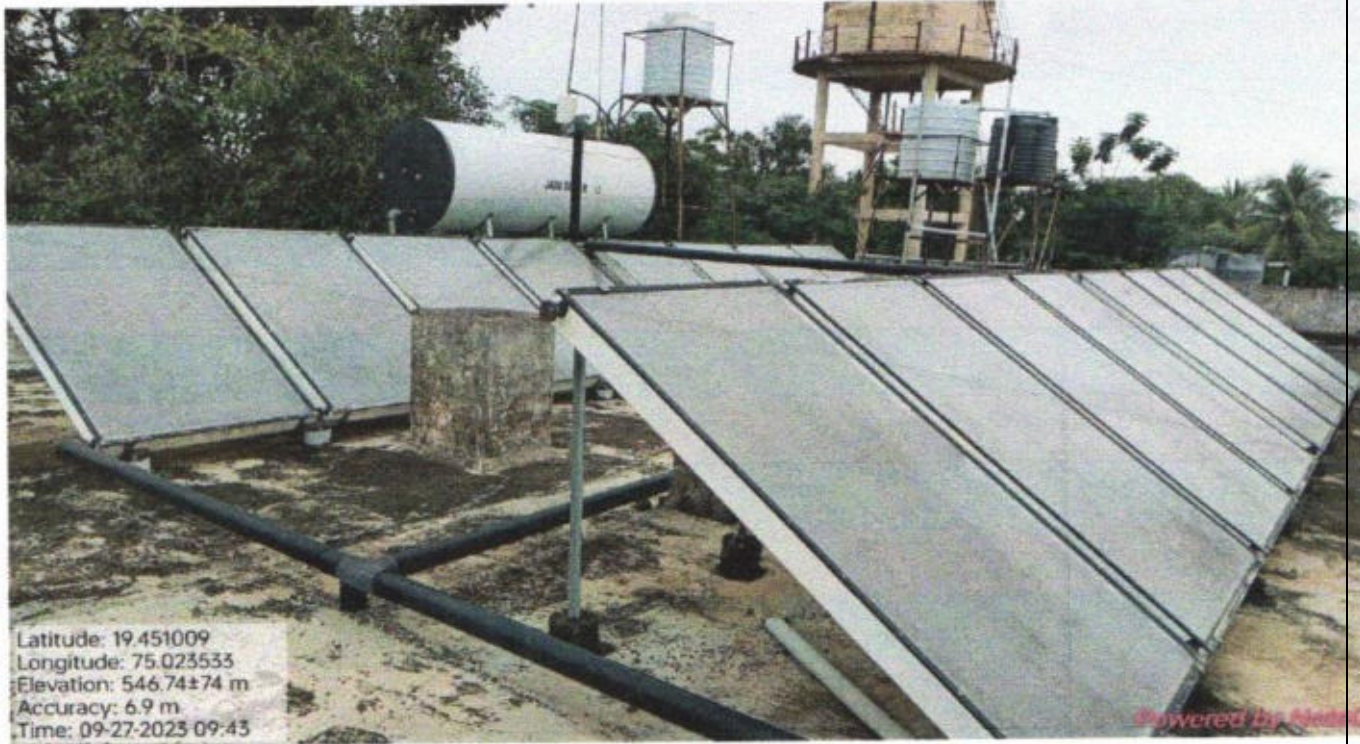
Jain Solar Water Heater System, close Loop 2000 LPD
